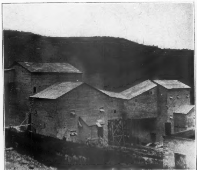
The Secondary Crushing, Screening and Storage Units
